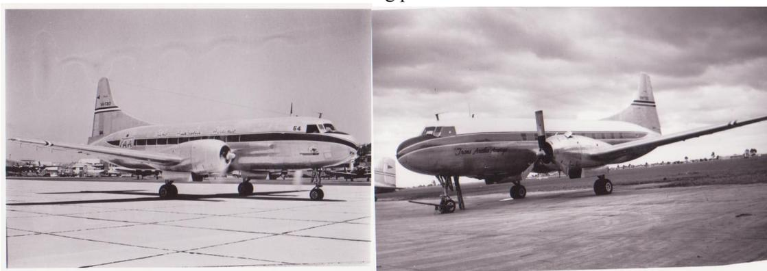
The one on the left is VH-TAQ on the tarmac at San Diego, all bright and highly polished and the second photo is in Melbourne after it was decided that the upper part was to be painted white to reflect the sun and reduce the heat inside the aircraft during turnaround. Note where the name *Trans-Australia Airlines* was painted on the initial aircraft, and it was later repositioned along the fuselage and above the windows.
